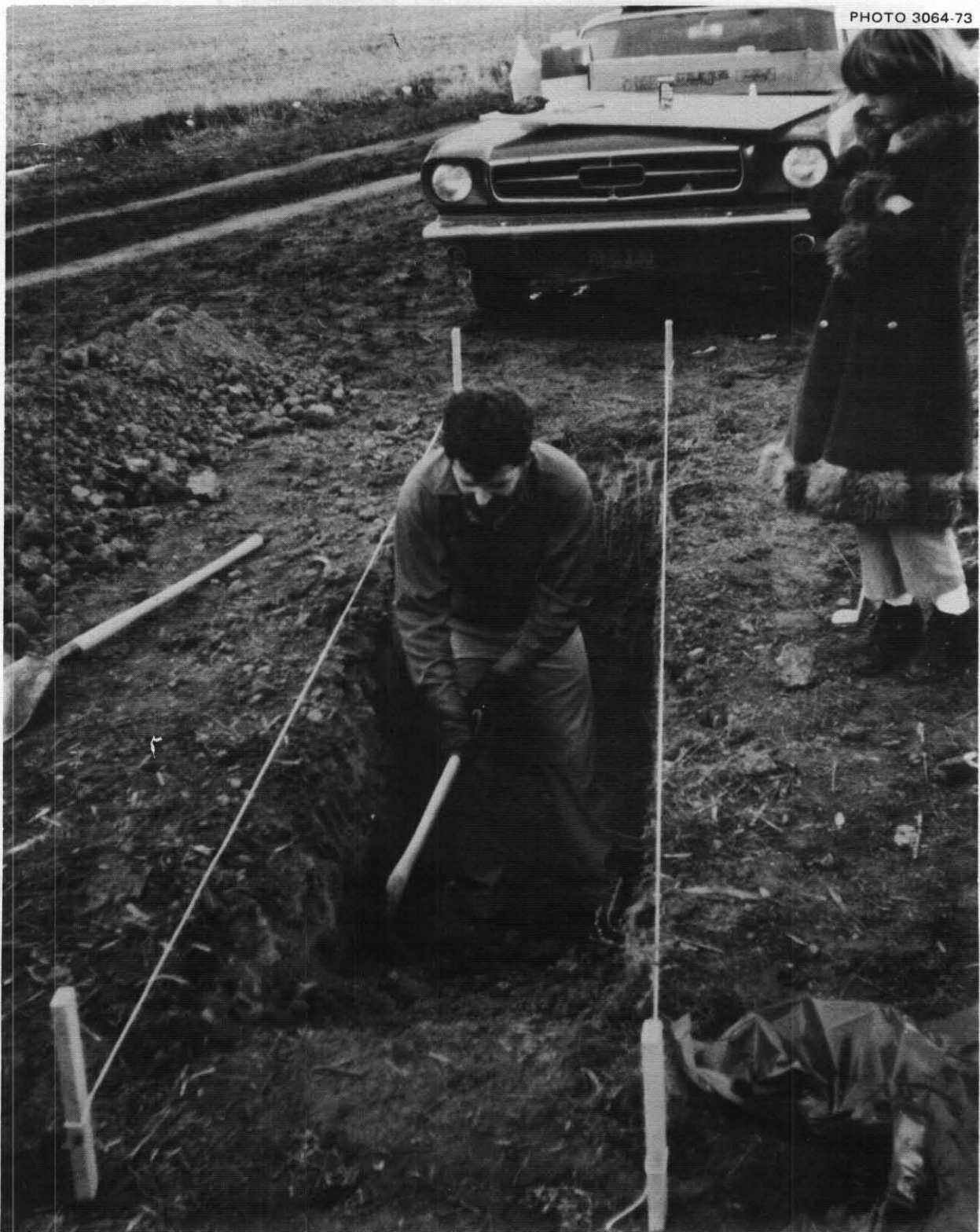
Fig. 6.6. The father swung his pick properly, a result of his learning to use an ax as a boy of 12, when his family spent a while in rural Oregon. However, he tied unnecessary strings between the stakes, and left them tied, and dug the trench too narrow. Later, he spent about two hours inefficiently widening it.
